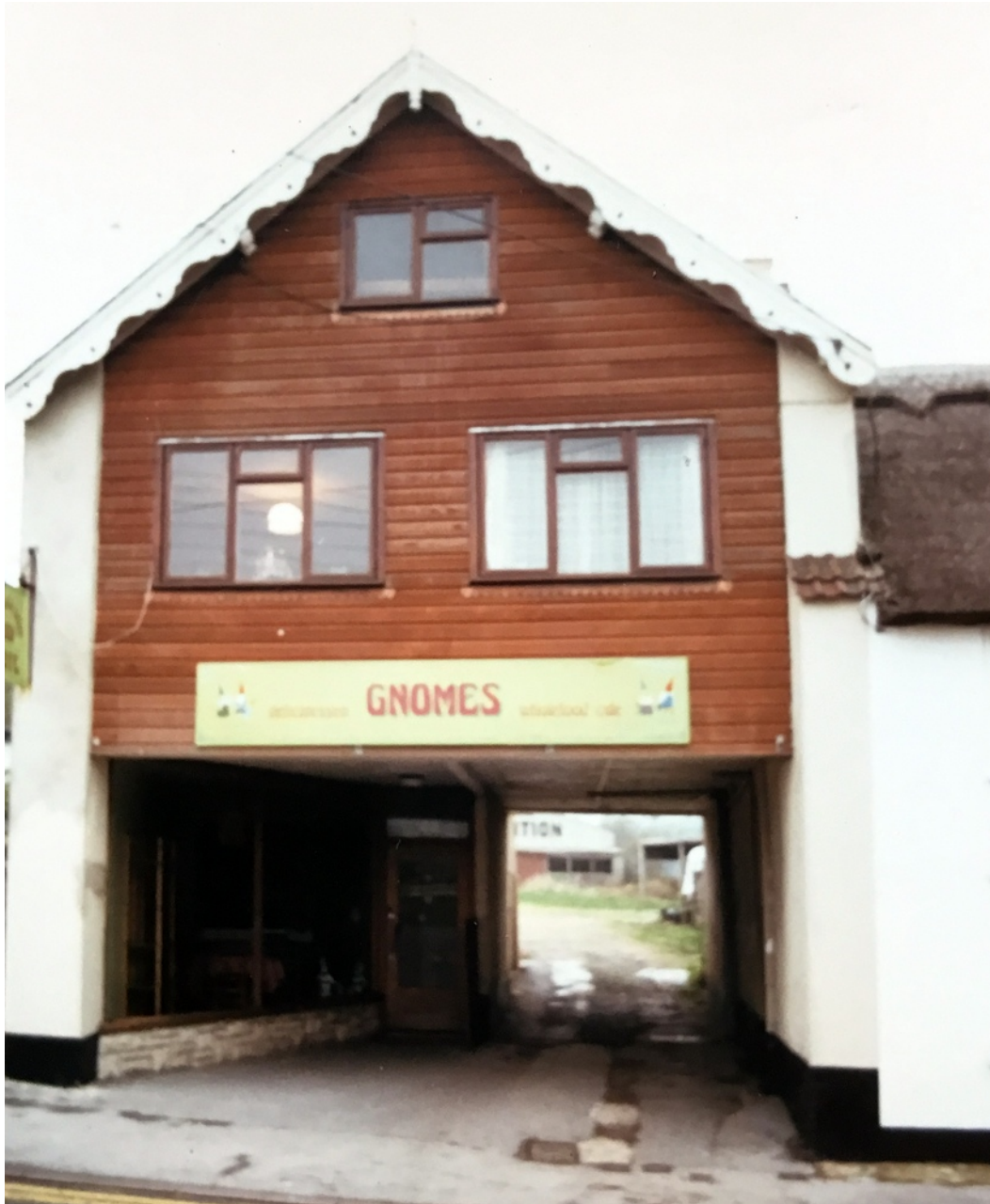
The building on the end of Firlands that was demolished to make access to Barneys Close in the 1980's
